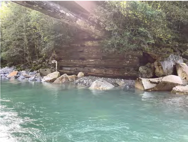
Right Bank Abutment when facing downstream
