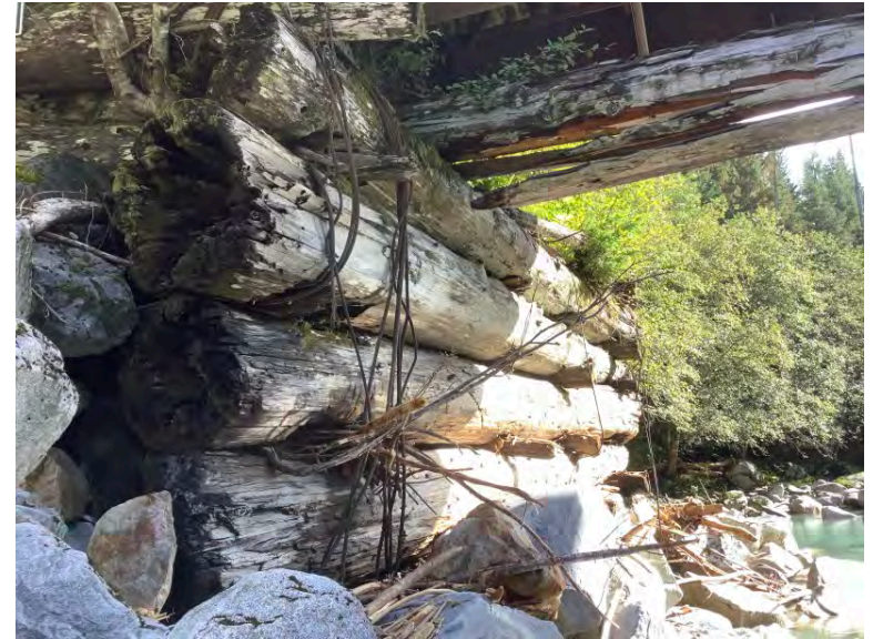
Left Bank Abutment when facing downstream
